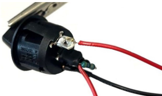
Fig. 10: Correctly soldered cable
